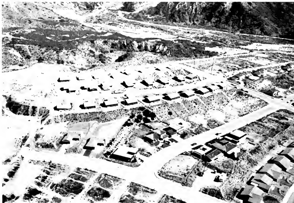
Photo 12. Houses being framed (photo 8) were located in top center; those partially completed in the left center and top left (photo 9); and those completed are in the foreground and far right (photos 10 and 11).
